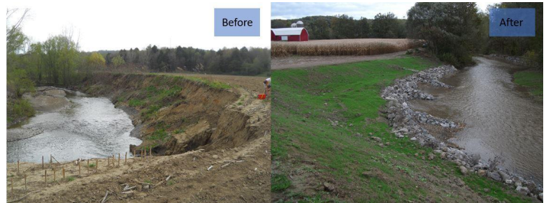
Streambank stabilization installed in Erie County, Pennsylvania using GLSNRP funding.
