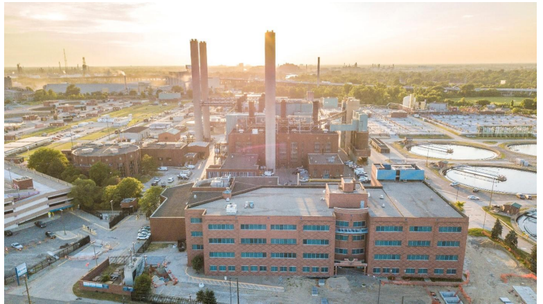
Great Lakes Water Authority treatment plant.
